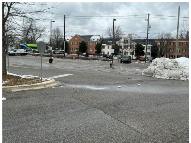
36 - PARKING LOTS / POLE LIGHT FIXTURES
