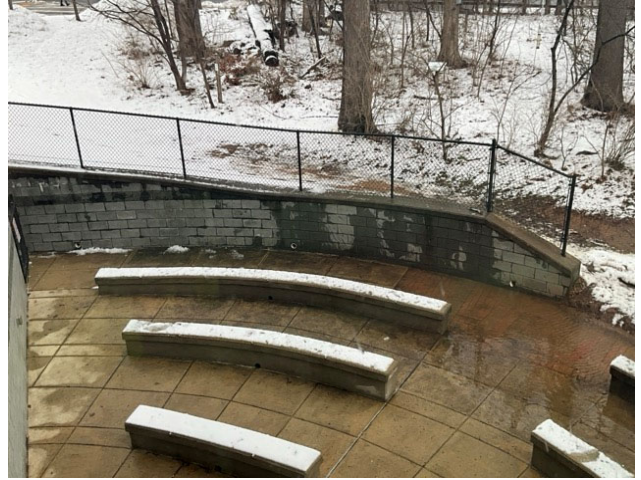
38 - RETAINING WALL / FENCING
