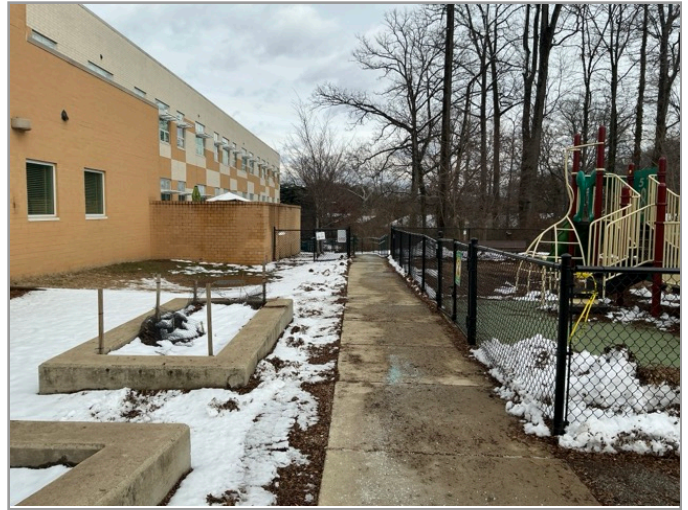
ACCESSIBLE ROUTE TO PLAYGROUND
