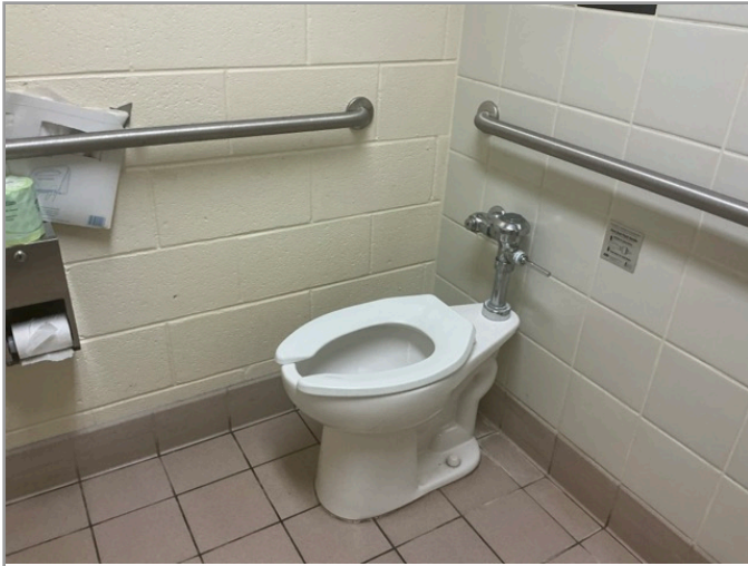
TOILET STALL OVERVIEW
